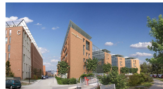
Infopark Budapest Building D
