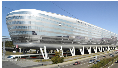
Airrail Center development project, Frankfurt
